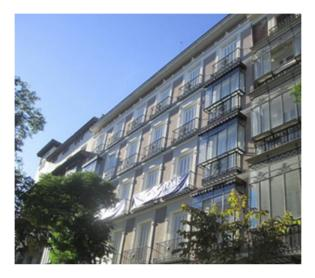
The building is located at N°6 in the Calle Salustiano de Olózaga in Madrid and dates back to the 19th Century and is a perfect example of the noble construction of this period: Load-bearing walls composed of a framework of studs and sleepers, braced with masonry brickwork and lime mortar. These walls were normally arranged parallel to the main façade, acted as supports to the wooden joist flooring which made up the five floors of the building.
