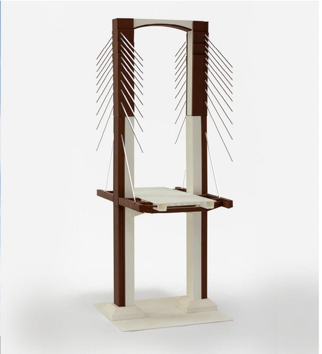
The Centenario Bridge in Seville shares a structural typology and cable technology with the Fernando Reigh Bridge in Alcoy. Both bridges of the State Highway Network employed the cable technique available at the time of their construction: prestressed strands embedded in cement grout confined in a black polyethylene outer sheath. The only difference between them being that a second outer sheath with a white finish was placed on the Centenary Bridge.
